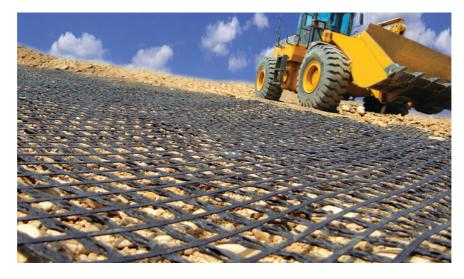
Requirements such as separation, filtration, drainage, reinforcement, tension equalisation and protection are becoming increasingly important in the construction industry. Warp knitted geogrids or geocomposites can be used here. The requirements for the physical characteristics of the textile substrates demand top-quality production methods in order to optimally exploit the properties of the high-performance fibres.
